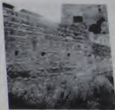
Fig. 245. S. Teodoro. One masonry wall of opus caementicium in detail.
